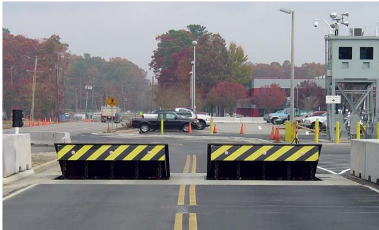
Figure 47: Vehicle Entry Point
