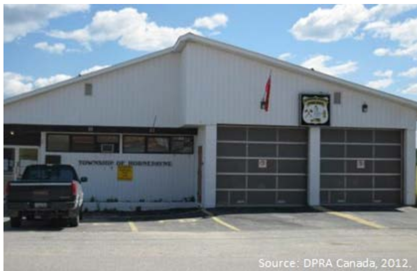
Figure 19: Township of Hornepayne Municipal Offices
