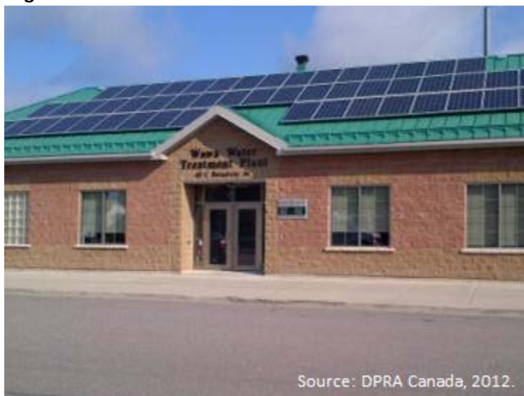
Figure 42: Wawa Water Treatment Plant
