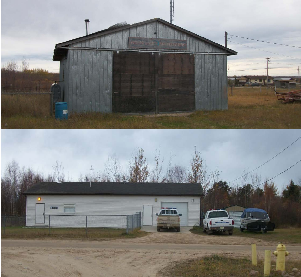
Figure 6-3: Fire Department and Police Station in English River First Nation, Patuanak
