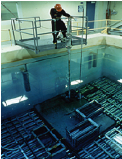
Figure 6-2 Example of Used Fuel Storage in Bays at Reactor Site
