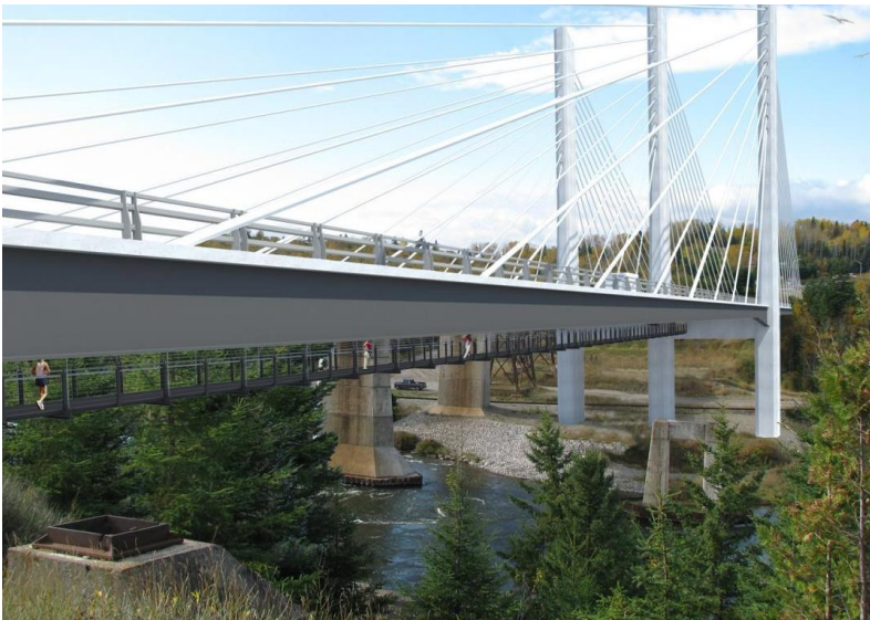
Figure 38: Conceptualization - Pedestrian Walkway of Nipigon Cable-Stayed Bridge
