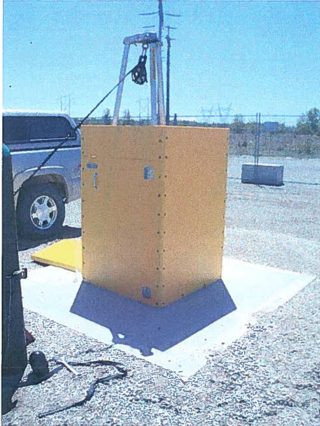
Figure 4. Example of concrete pad with well head enclosure and temporary test equipment
