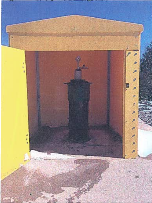
Figure 3. Example of an enclosure placed atop of the instrumented well head.
