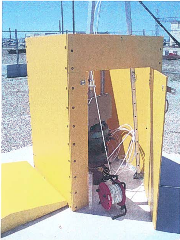
Figure 5. Example of well head enclosure and temporary test equipment
