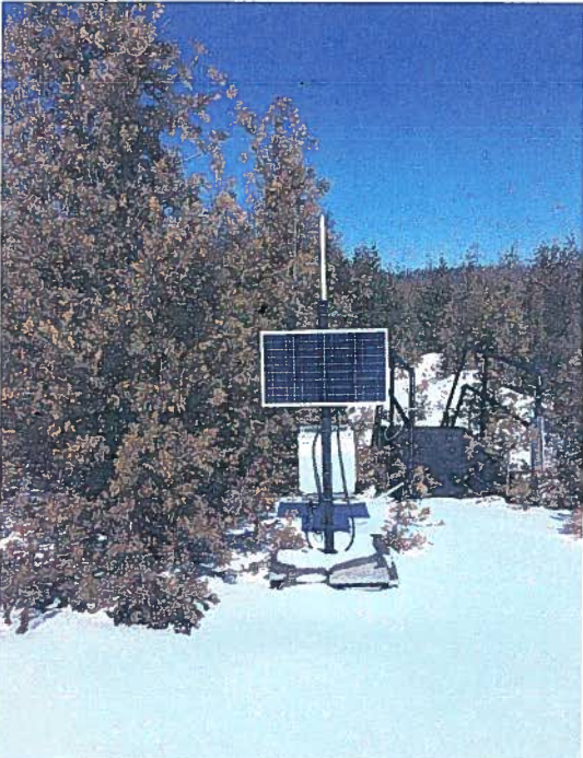
Figure 6. Example of a solar panel, battery and data transfer equipment (in addition to the well head enclosure)
