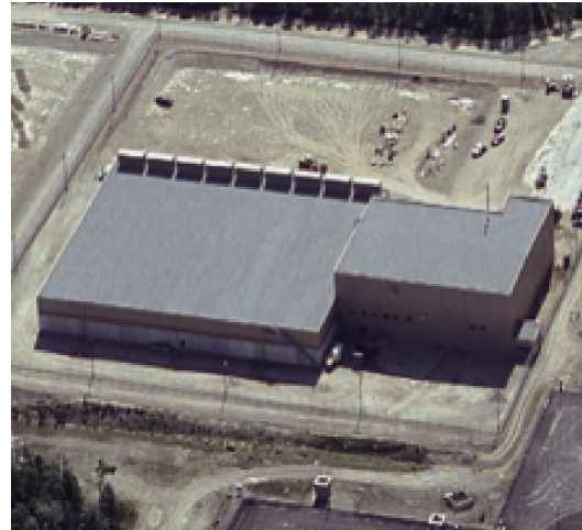
Figure 6-3 & 6-4 Example of Used Fuel Storage in Dry Storage at Reactor Sites – Surface Storage Building and Dry Storage Containers
