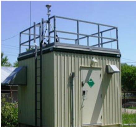
Air quality monitoring station
