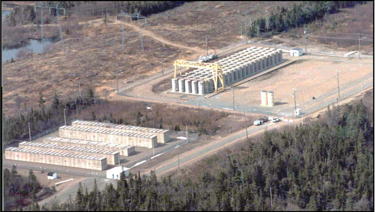
Figure 6. A Typical Spent Fuel and Radioactive Waste, Surface-Storage Facility in Canada. The Cylindrical Concrete Canisters in the Background (100 of them) are sufficient to safely hold the approximately 1000 Tonnes of Spent Fuel from about 10 Years of Full Power Operation of a CANDU Reactor. The Site will accommodate 200 more such Canisters to securely contain all Spent Fuel from at least Thirty Years of Reactor Operation. The Concrete Structures in the Foreground hold relatively low to moderate dose rate Maintenance and Process Wastes. (Photo, Courtesy of NB Power).
