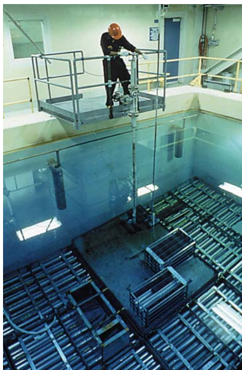
Figure 2.1: Pool Storage at Pickering
