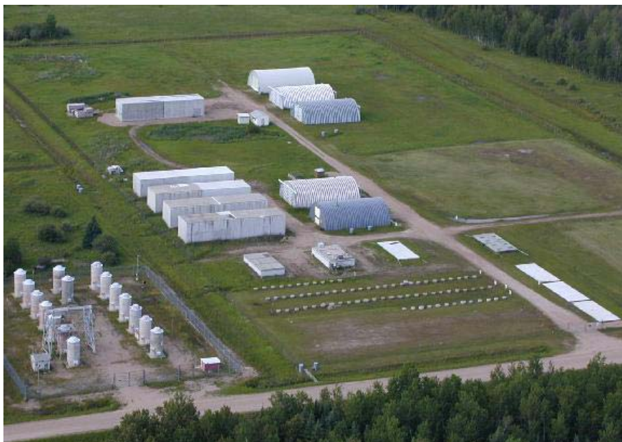
FIGURE B-1 WR-1 USED FUEL STORAGE
