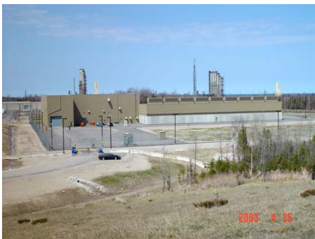
Figure 2.6: Western Used Fuel Dry Storage Facility
