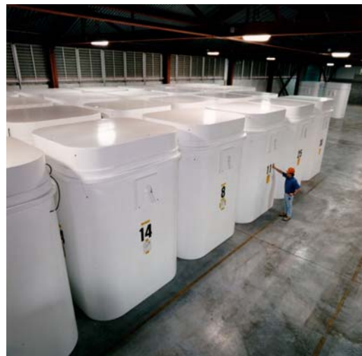
Figure 2.2: DSCs in a Storage Facility
