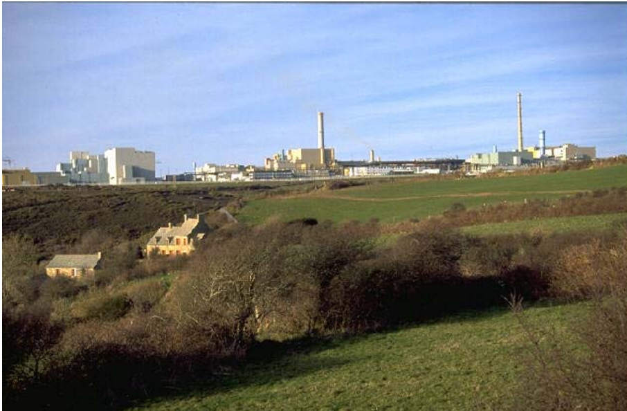
Figure 8 Reprocessing plant at La Hague France (COGEMA Archives/Phillipe Lesage)
