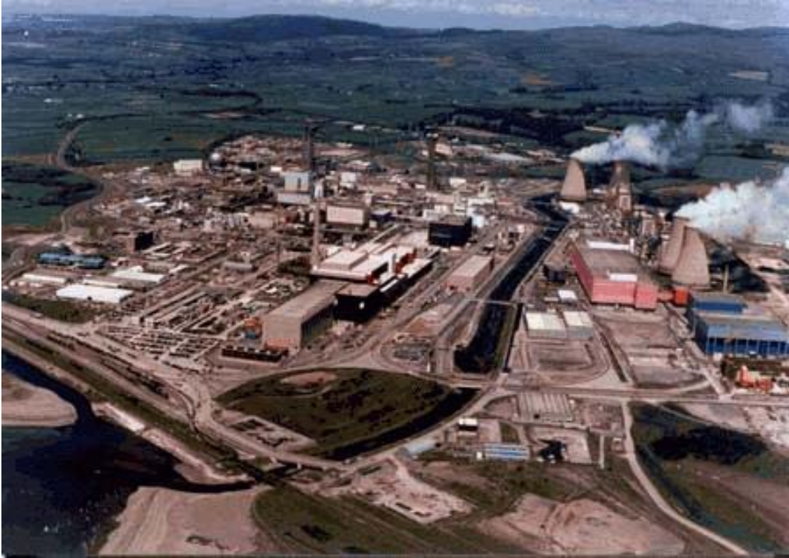
Figure 7 Sellafield nuclear complex in the UK. The THORP facility is in the large complex with the white roof in the centre of the photograph (by permission British Nuclear Fuels Limited)
