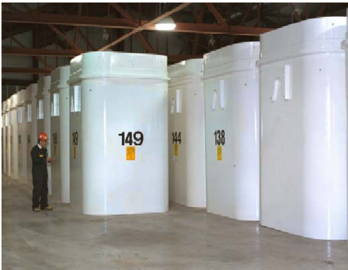
Figure 3. Concrete Dry Storage Containers with 10-year cooled used fuel. (“Pickering Waste Management Facility Phase II Information Package”, OPG).
