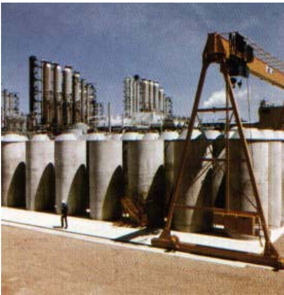
Figure 1. Douglas Point fuel storage silos, Ontario, ( www.nuclearfaq.ca/drystrge.htm )
