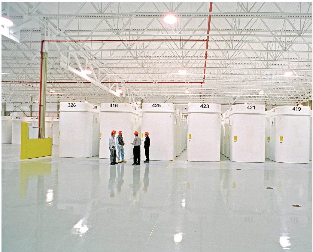
Figure 2: Dry storage casks at OPG’s Western Waste Management Facility, Tiverton, Ontario
