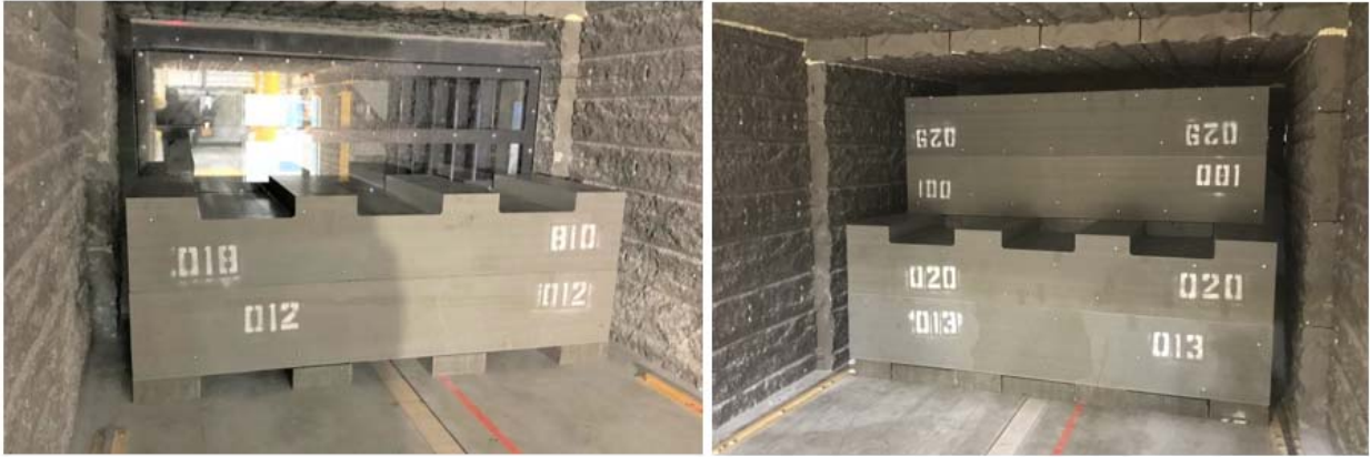
Figure 7.13: Buffer Boxes in Placement Room
