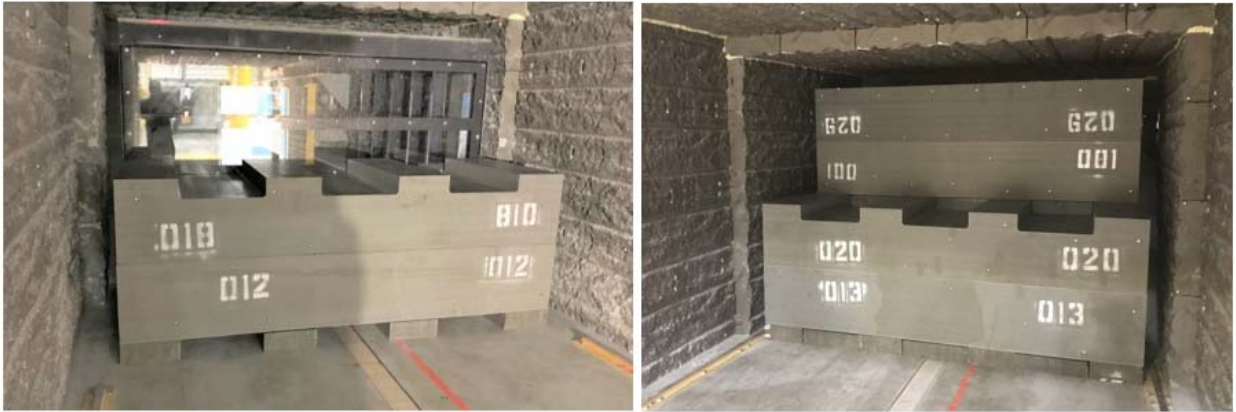
Figure 7.13: Buffer Boxes in Placement Room
